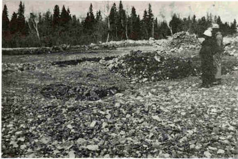
Figure 7: Photo of Sinkhole in Glacial Fluvial Sands Over the 119 Area
